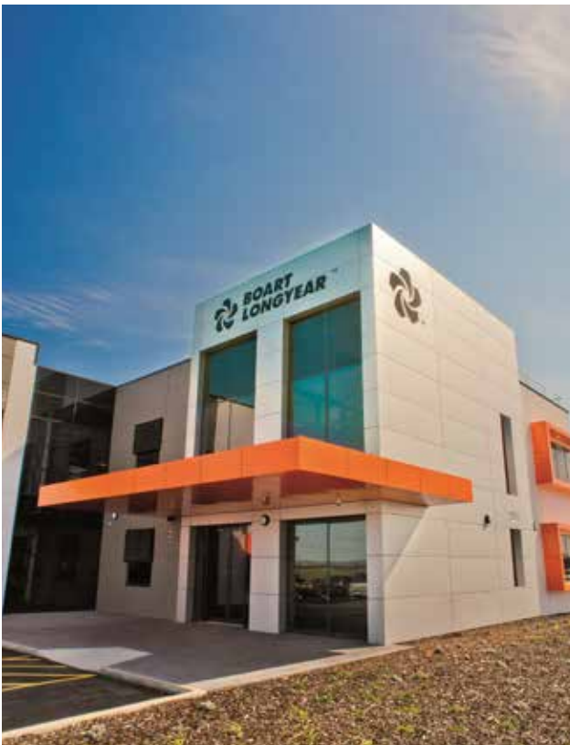
Figure 11.1 Boart Longyear building within the Burbridge Business Park Policy Area
